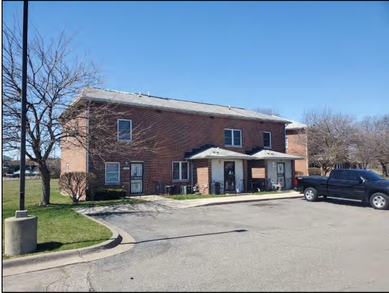
Photo 21: Parkside Homes Apartment Building 12054-12058, built 1938, facing northwest.
