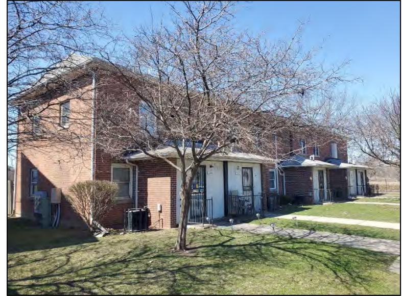
Photo 22: Parkside Homes Apartment Building 12060-12068, built 1938, facing northwest.
