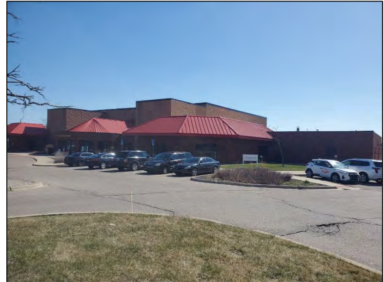
Photo 4: 5405 Conner Street, built 2010, facing east.
