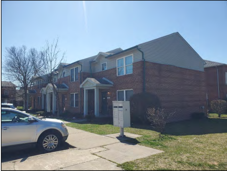
Photo 17: Parkside Homes Apartment Building 12232, built c. 1998, facing south.
