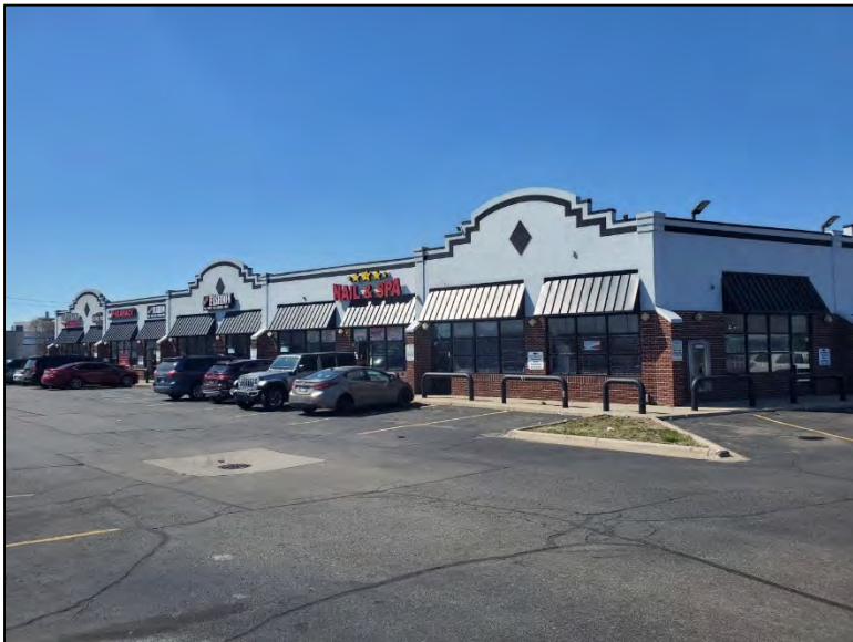
Photo 7: 11919 E Warren Avenue, built 2001, facing southwest.
