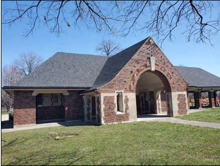
Photo 9: 12200 Chandler Park Drive, built c. 1920, facing east.
