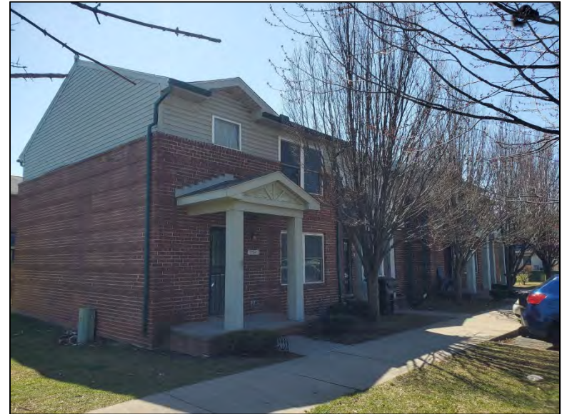
Photo 16: Parkside Homes Apartment Building 12246, built c. 1998, facing south.
