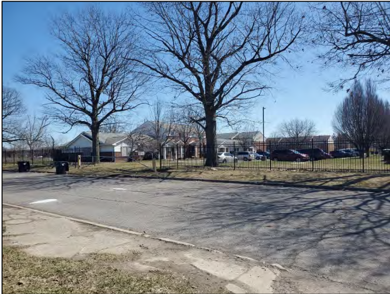
Photo 23: Overview of apartment buildings in the APE from Frankfort Street, facing southwest.
