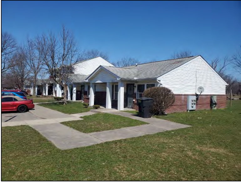
Photo 13: Parkside Homes Apartment Building 12330, built c. 2000, facing north.
