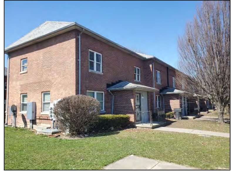
Photo 14: Parkside Homes Apartment Building 12318, built 1938, facing northwest.
